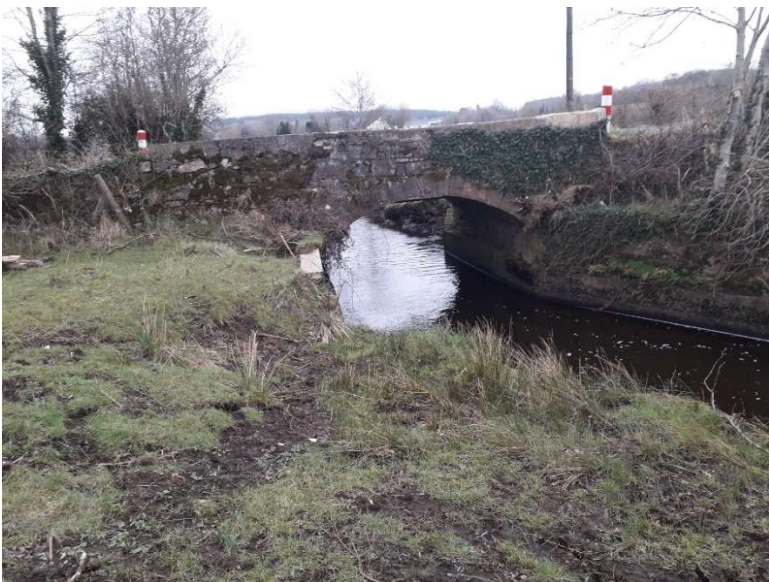
Figure 8 - Bridge 3 located along R4230.
