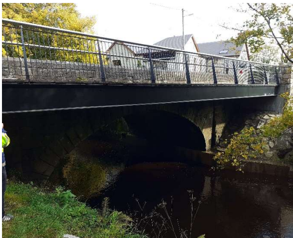
Figure 3 – Extended walkway attached a bridge.
