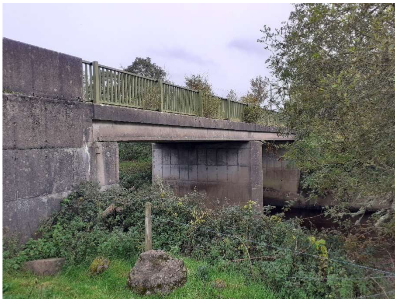
Figure 2 - Bridge structure within L4165 crossing Bonet River (Lough Gill SAC & pNHA)
