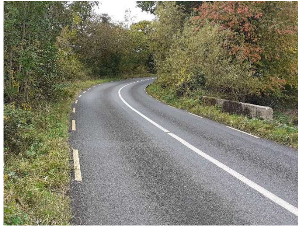
Figure 5 – Bridge 7 located within R287 with sweeping bend.
