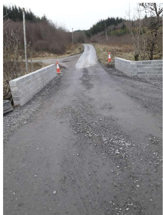
Figure 9 - Bridge 4 situated north of proposed SS location.
